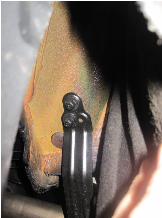
Picture 7 – Behind the inner rear fender liner
